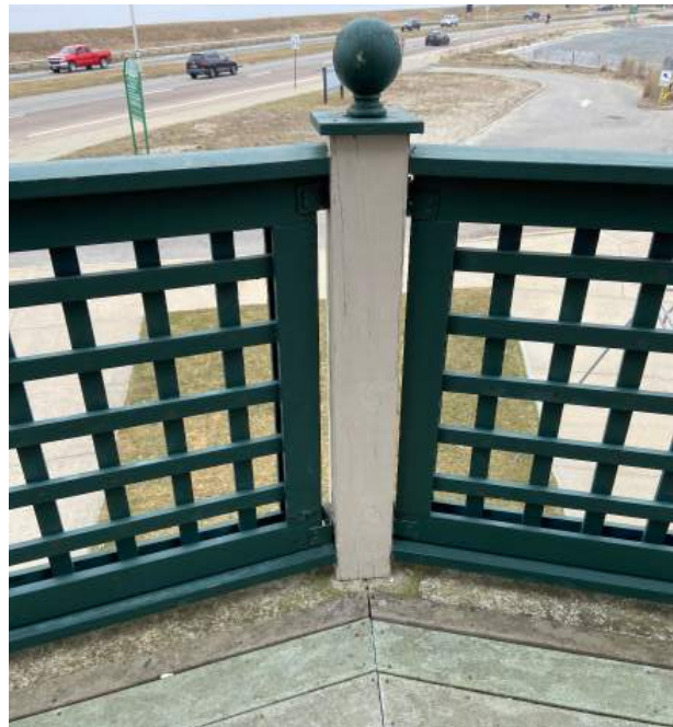
60. Typical railings along the edge of walkways and decks.
