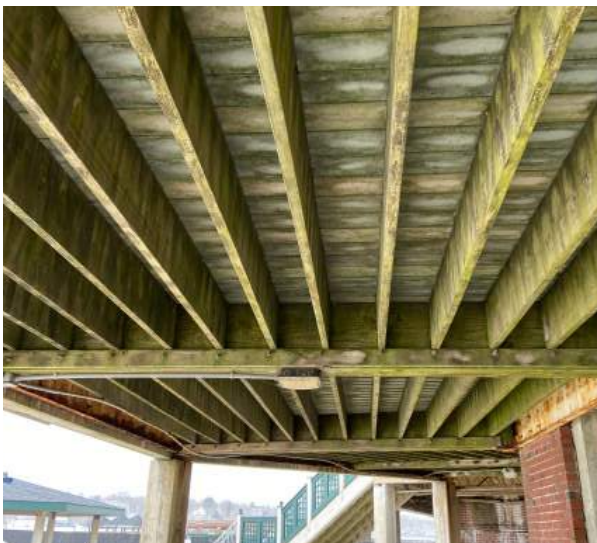
52. Ledgers supporting the edges of deck boards.
