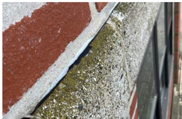
19. Rubber, flexible-type flashing at window head.
