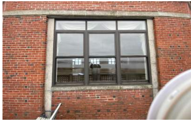
18. Window from exterior.
