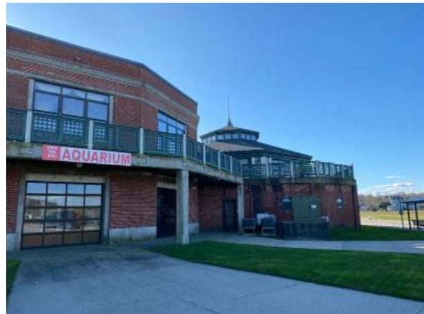
10. Rotunda (left) and Carousel Building (right) from the north.
